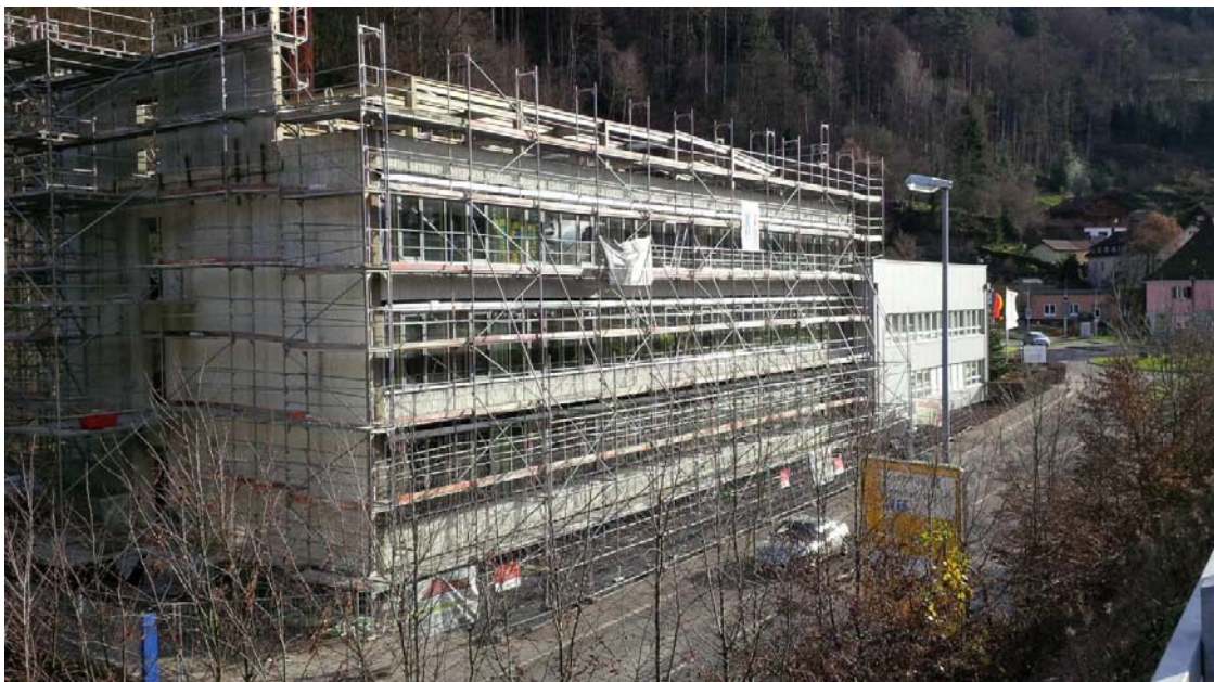
New Research/Development, Sales/Marketing and Administration Building (under construction January 2014)
